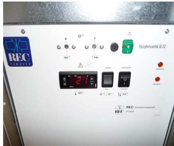
Figure 38 Air treatment system unit for a single apartment, used in building D.
