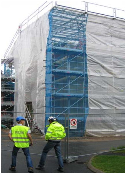
Figure 3.7 and 3.8 Protecting a building site and stored materials often pays back as improved work efficiency even though the main purpose is to avoid moist/damp construction parts and mould growth.
