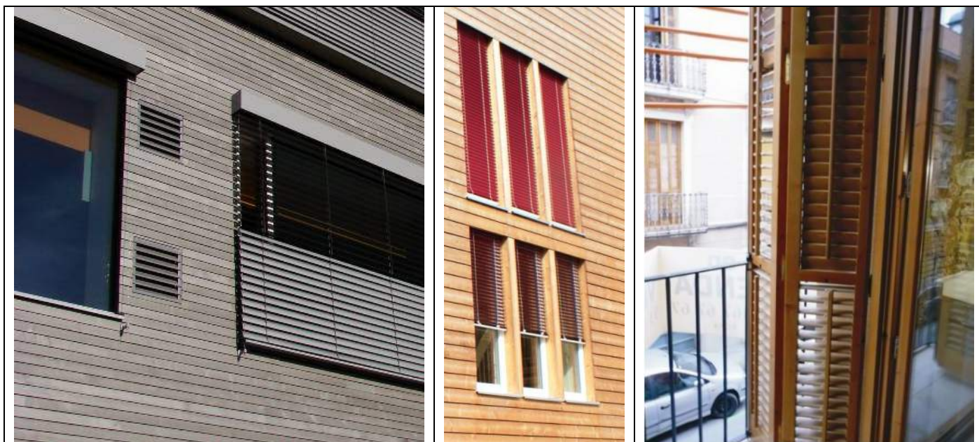
Figure 9. Two examples of external shading with outside blinds; the left picture shows light directing blinds - the upper part of the blind directs daylight into the room (Reference: AEE INTEC)
