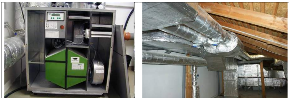
Figure 18. Ventilation device with integrated heat recovery and insulated ventilation pipes (References: AIT; AEE INTEC)
