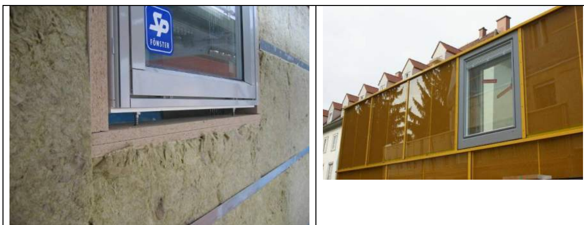
Figure 6. Three pane windows with an U-value of 0,85 \text{ W/m}^2\text{K} , used in the pilot project Brogården/Sweden (left picture) and module-integrated passive house windows at Dieselweg Graz/Austria (References: SP and AEE INTEC)
