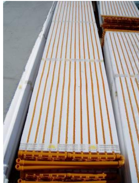
Picture 4: Wall heating system used between old and new exterior wall at Dieselweg, Graz; AEE INTEC
