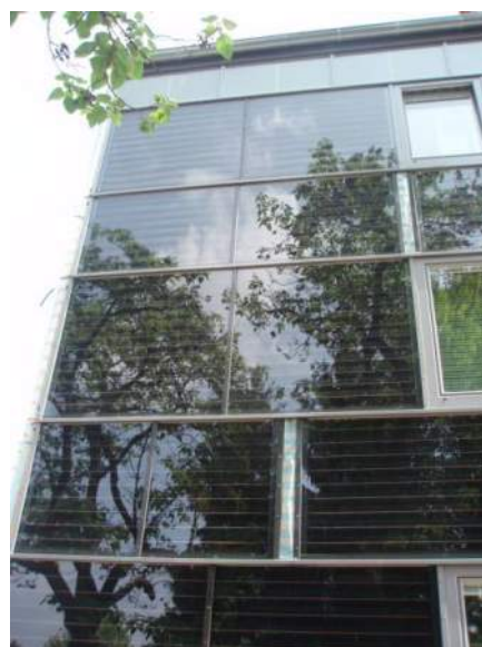
Picture 5: Solar thermal façade collectors at Dieselweg, Graz; AEE INTEC
