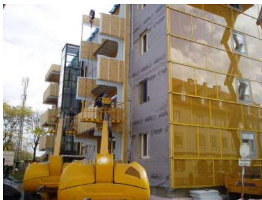
Picture 2: Pre fabricated and insulated modules at Dieselweg, Graz; AEE INTEC
