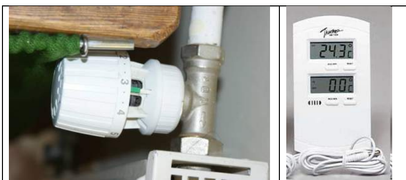
Figure 17. Thermostatic valve and outside temperature sensor (References: AEE INTEC; Star)
