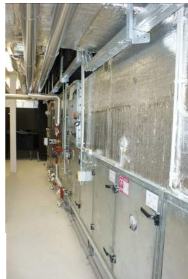
Picture 7: Big ventilation device with integrated heat recovery; AEE INTEC
